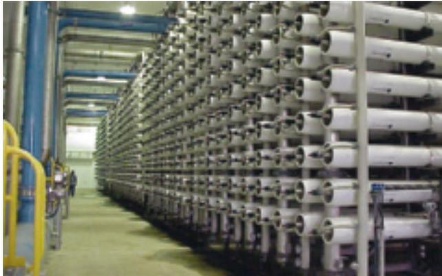
**Figure 1.10** Seawater reverse osmosis membrane filtration installation in Larnaka, Cyprus. The permeate production capacity is 54,000m<sup>3</sup>/day. The total amount of eight-inch diameter membrane elements is 5,800. The plant size can be estimated from the person shown on the left of the figure
