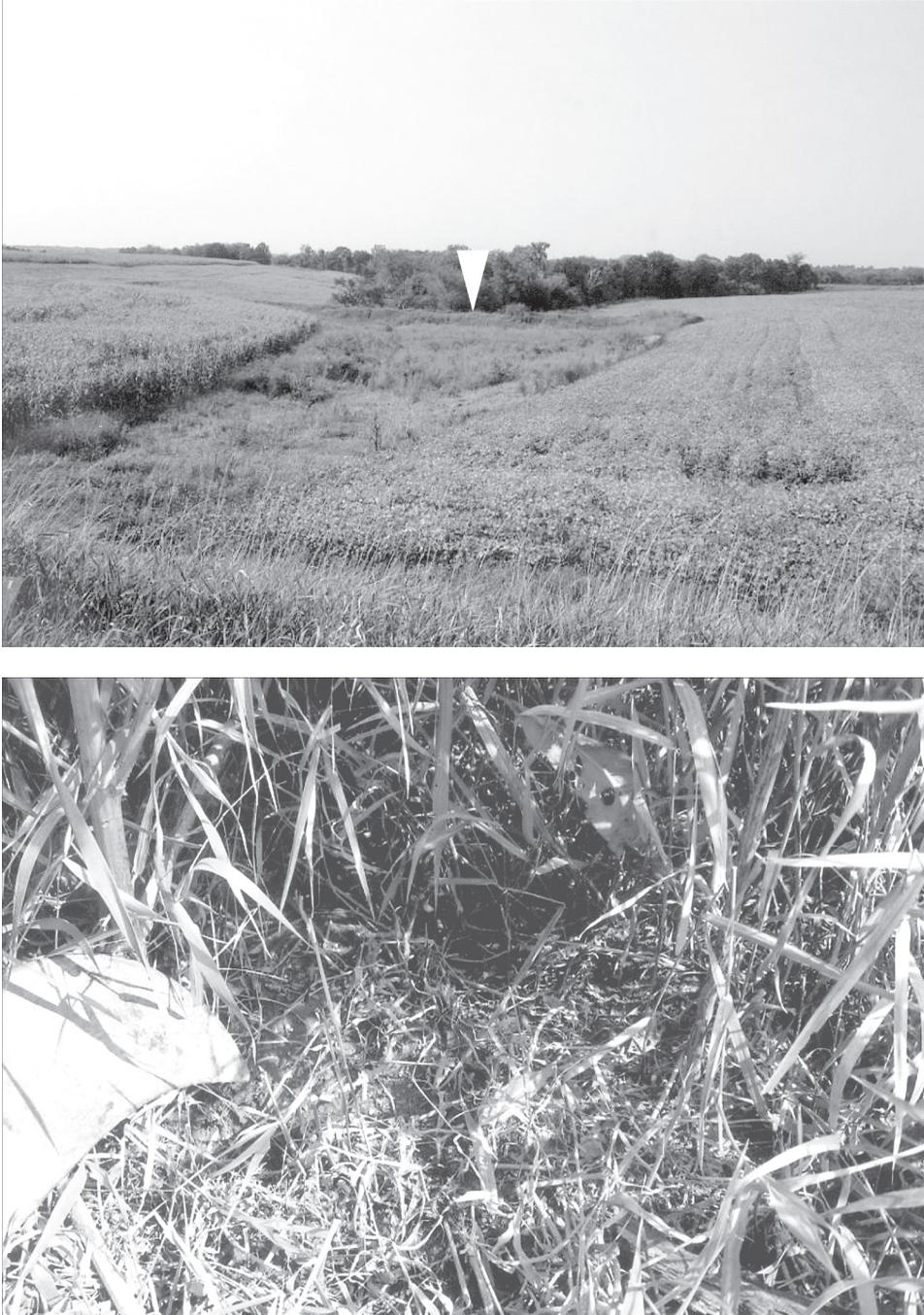
**Figure 8.4** A sediment trap after the 2007 storm. Top: A “dry” floodwater retarding dam (arrow) controlling about 8–10 acres (3–4 ha) of mostly no-till crops, 5 mi (8 km) north of Altura, MN, on Beaver-Altura Road looking west. P = 10 in. (25 cm). Corn is to the left and soybeans are to the right. Bottom: Bottom of dry pond. Note lack of any sediment accumulation. NW1/4, Sec. 19, T18N, R9W, Winona County, MN. Photos made Sept. 2–9, 2007.
