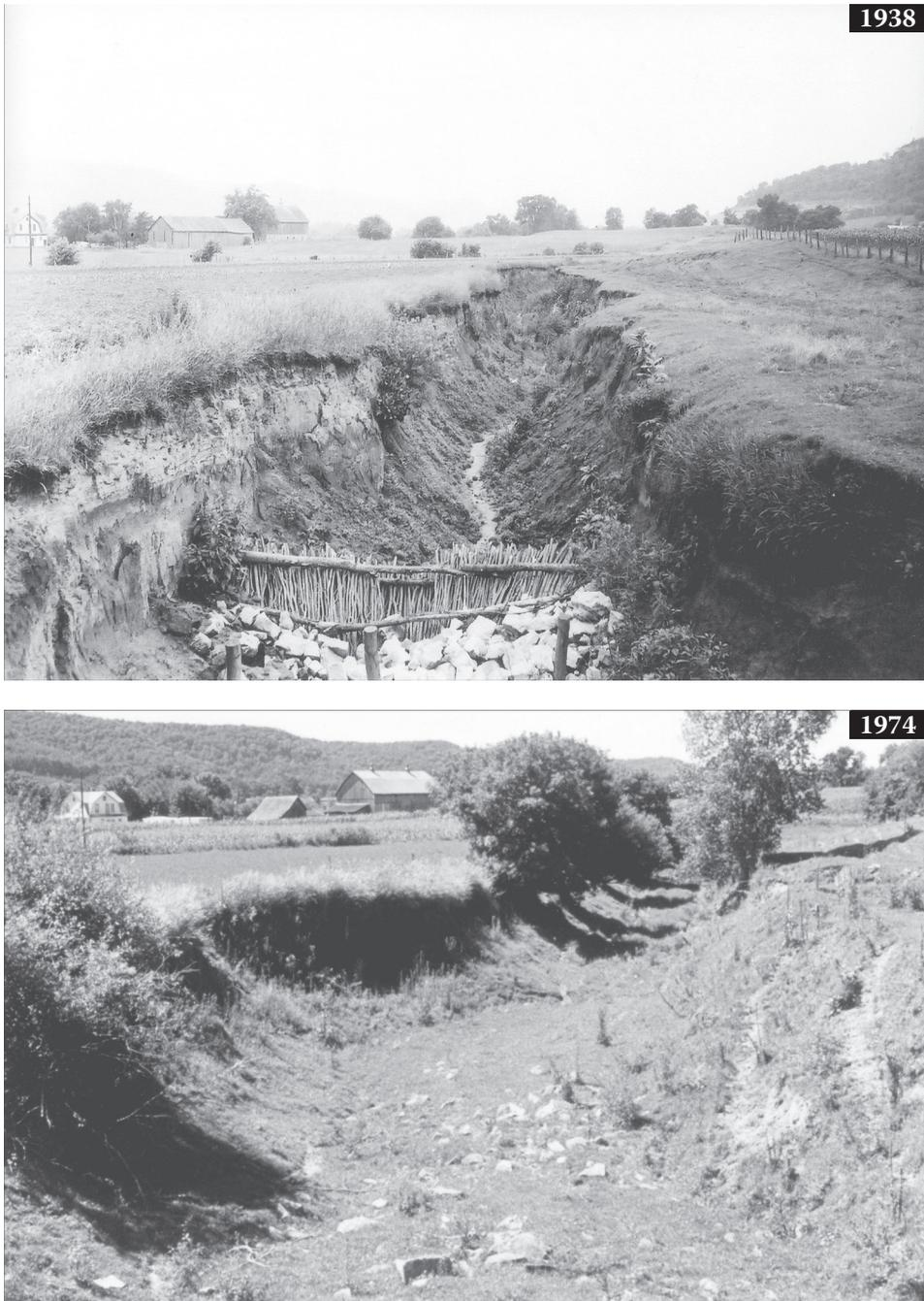
**Figure 8.9** Gully 1 mi (1.6 km) north of Chaseburg, WI, looking downstream from bridge on County K, P > 12 in. or 30 cm (SW1/4 Sec21 T14N R6W, Vernon Co.). Top: July 1, 1938. Note about 3 ft (1 m) of light-colored, historical sediment accretion on bank and apparent recentness of gully incision. A storm the next day destroyed the timber and rock revetment. Photo by S.C. Happ. Bottom: 1974. Note that gully more than doubled in size after 1938 but was stable by 1974. (Continued)
