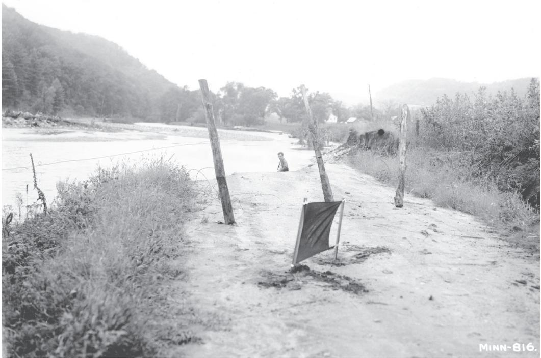
*Figure 5.6* Fairwater, road from Elba to Fairwater about 1 mi east of Fairwater, 9/38, looking west. Several hundred feet of roadway eroded away.
