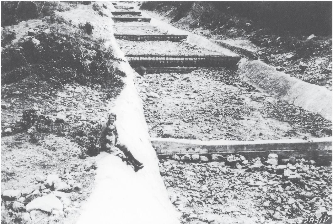
*Figure 4.9* Examples of elaborate drop structures to control hillside gullies creating rock fans on transportation routes. Top: Near Genoa, WI, to protect railroad, 6/27/30. Bottom: Between Wabasha and Lake City, MN, 1932. (Photos credit: C.G. Bates.)
