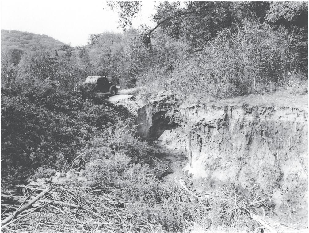
**Figure 4.2** Gully heads (overfalls) threatening economic activity in the late 1930s. Top: A threatened farm possibly in Trempealeau Co., WI. Bottom: A threatened roadway in Wabasha Co, MN, 2 mi (3 km) SW of Weaver.
