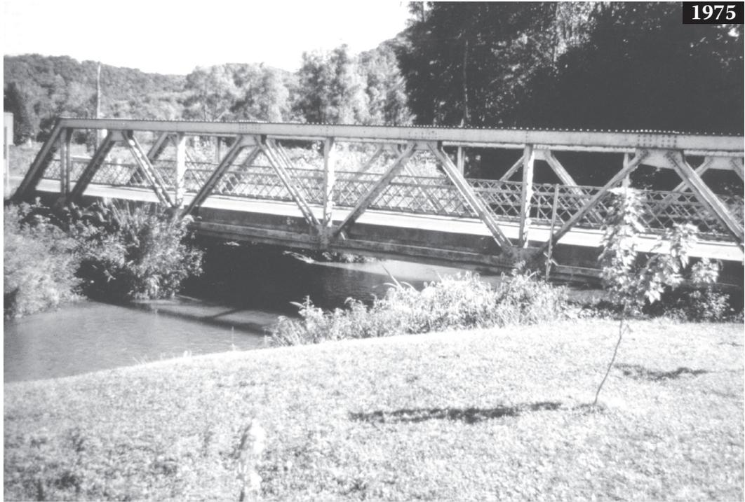
*Figure 7.4 Continued* 1975: Replacement bridge at the same site as above, looking southeast (upstream). The newer bridge sat about 1 ft (30 cm) higher than the old bridge but had only about 4 ft (1.2 m) of clearance above the water in 1977. The 2011 water level here is 10–12 ft (3–4 m) higher than in 1914.
