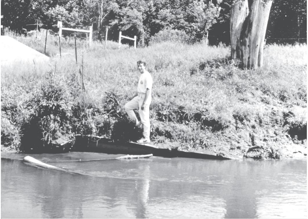
**Figure 7.23** The south abutment of an old Dodson Hollow Road bridge over Coon Creek (SE1/4, Sec 22, T14N, R6W, Vernon, Co., WI). This bridge was replaced in 1926 as the creek rapidly aggraded, and the abutment was later buried in the floodplain. When built, probably in the early 1900s, this abutment was at least 10 ft (3 m) above the water. A small lateral shift by the stream in 1993 exposed the old abutment. The newest bridge (c. 1990) is seen to the far left.
