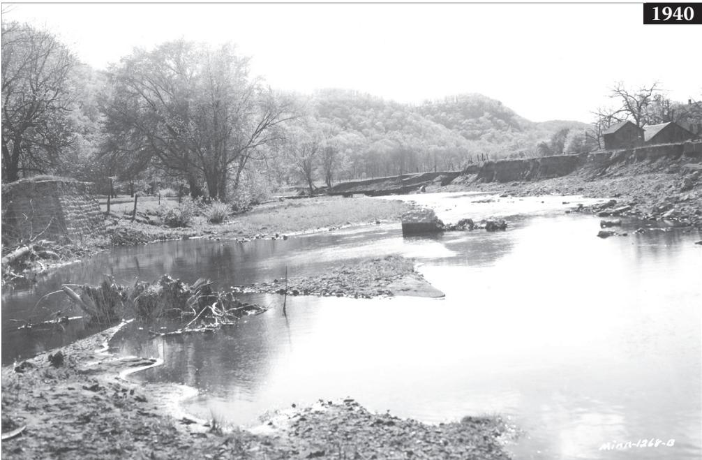
*Figure 5.5* Fairwater, bridge crossing visible in 5.1 and 5.2 looking upstream. c. 1905: the structure is probably slightly later than the one visible in 5.1 and 5.2 but is at the same crossing. Note stability of stream and banks. 1940: stream widened by about three times here so that right pier is near the center of the widened stream. The left pier is still visible (2006) in the village, but the recovering (narrowing) stream has buried the right pier in the new bank.
