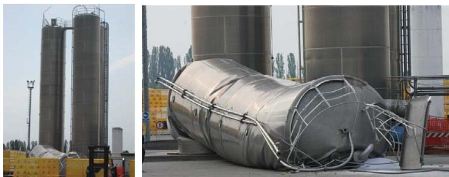
**Figure 1.** Total collapse of a slender silo during the earthquake series in Emilia Romagna/Northern Italy in 2012.
