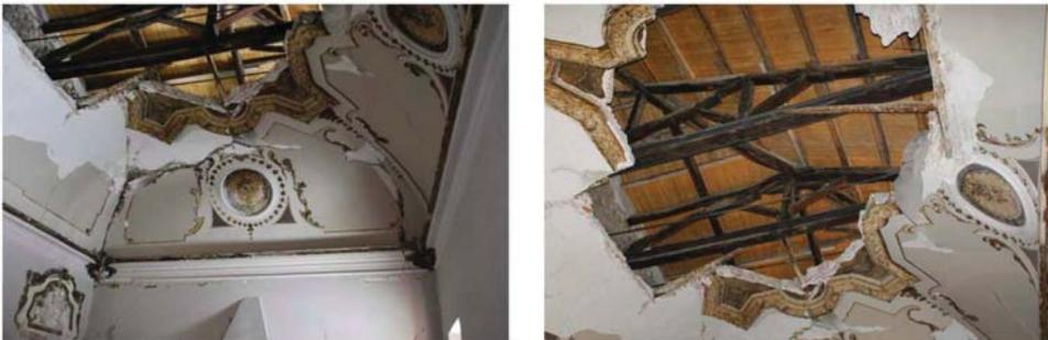
Figure 16. Pictures of the partially fallen vault.
