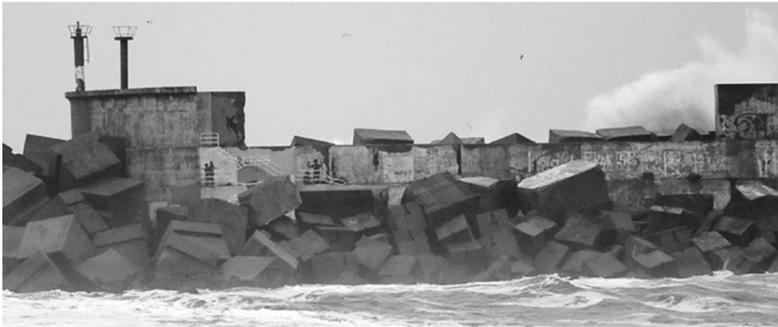
**Figure 18.** Displacement of the upper part of the crown wall in the breakwater of A Garda, Spain (2017).
