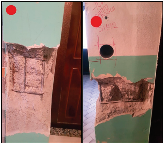
Figure 5. Column damages of a building to be demolished. Photos were provided by the study participant upon request of the authors. The intensity value provided by the participant was “Strong”.
