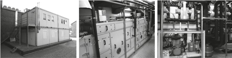
Figure 1. Test facility, air handling unit and heat pump with parts of the header system.
