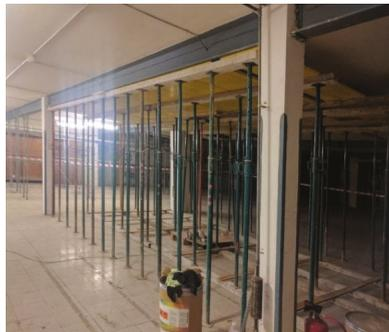
**Figure 8.** General view of the shoring and formwork on basement level -2 for safety reasons.
