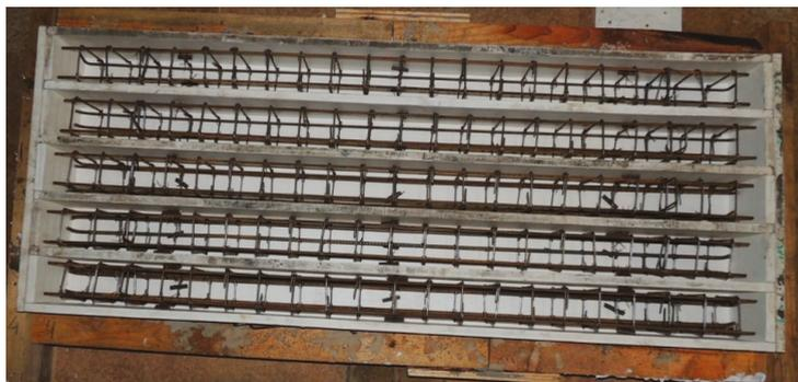
Figure 1. Beams before casting.
