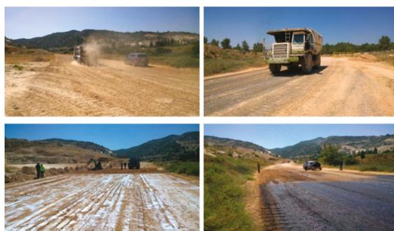
**Figure 4.** Application of the dust control product on the unpaved haul road before the dust emission experiment.
