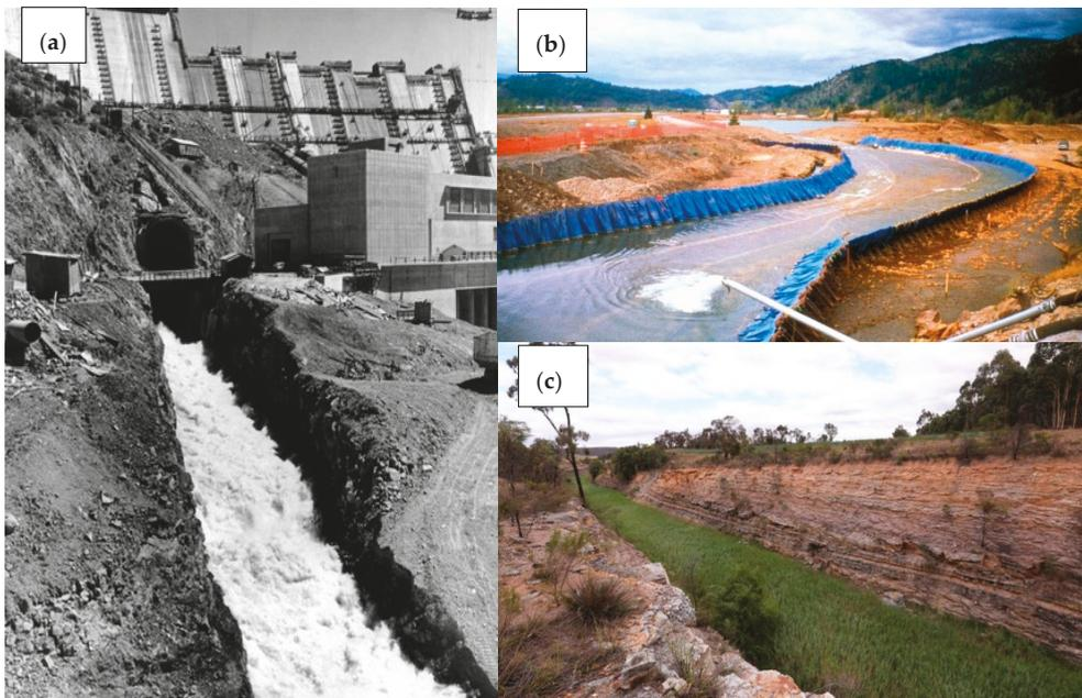
**Figure 2.** Examples of river relocation channels. (a) River relocation for the construction of the Shasta Dam on the Sacramento River (1943) (Photo: California State University); (b) the temporary relocation of the Coeur d'Alene River, Idaho, to allow the clean-up of contaminated tailings; (c) permanent river diversion of the Goulburn River for coal mining in NSW, Australia (Photo: Cathy Toby).
