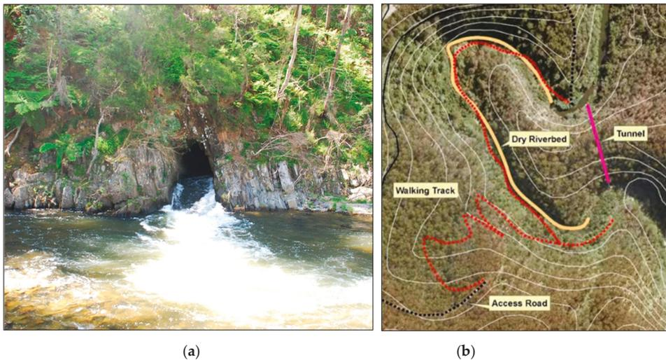
**Figure 7.** (a) Thomson River relocation, also known as Horseshoe Bend [62] (Source: Victorian Heritage Database); (b) diagram of residual reach and relocation tunnel (Source: West Gippsland CMA, 2010).
