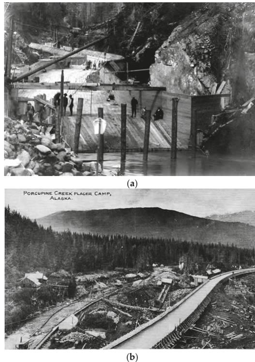
**Figure 4.** River relocation flume (circa 1907–1918) in the Porcupine Mining District, Alaska. (a) The flume was 2.4 km long, up to 2.4 m deep, and 7–12 m wide; (b) early flumes were prone to failure during floods (Source: Sheldon Museum).
