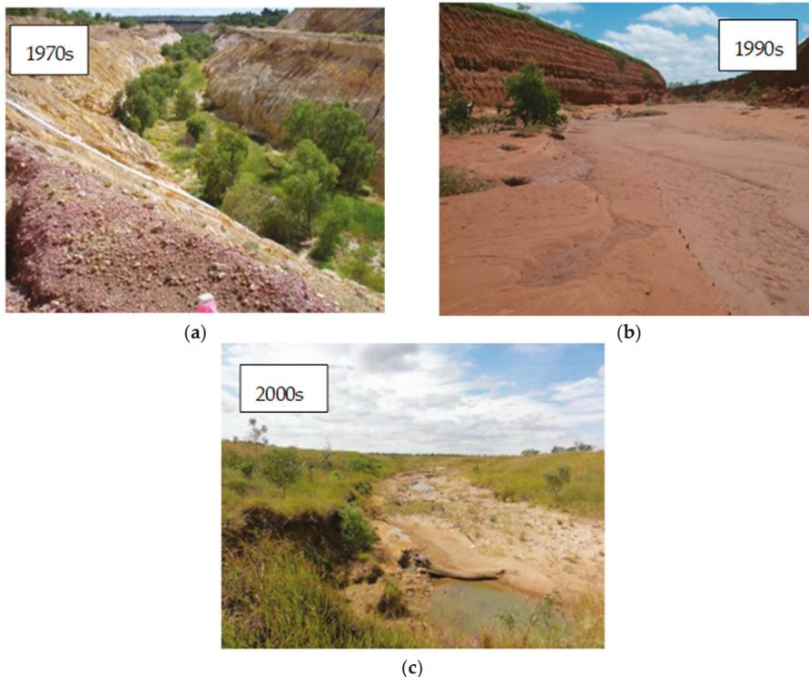
**Figure 9.** Changes in the design of relocated channels over time in the Bowen Basin, Queensland: (a) 1970s river relocation with a trapezoidal design and exposed banks; (b) 1990s river relocation with limited vegetation establishment, increased channel dimensions, and rill erosion on batter banks; (c) 2000s river relocation with a more natural bank batter and more natural morphology in the bed [69,70].
