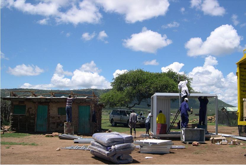
**Figure 36:** On-site construction of a Solarkiosk.
