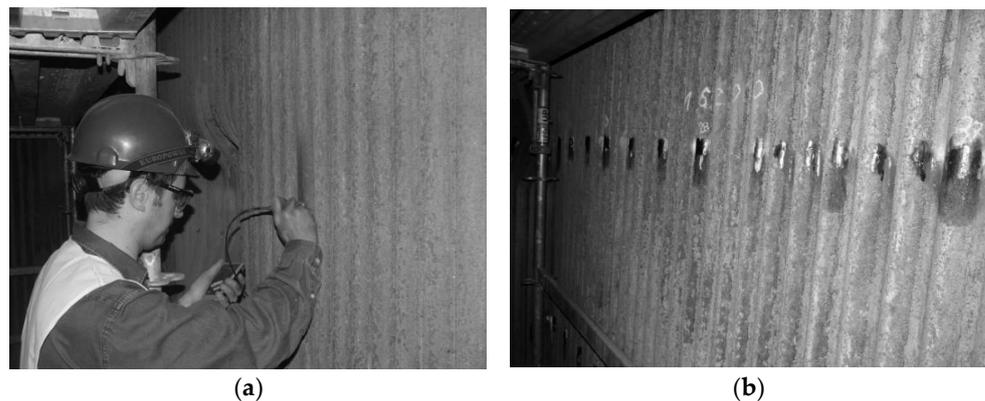
**Figure 4.** Measuring the tube thickness in the boiler with the aid of the ultrasonic method: (a) the measurement process; (b) the measurement points.
