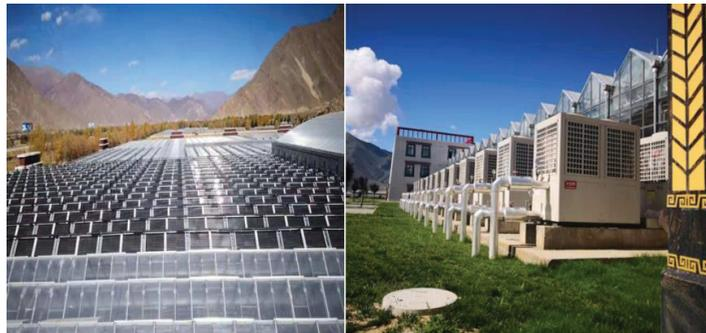
**Figure 14.** Overview of the Solar + Water Source Heat Pump Heating Project of Caina Township Government [114].
