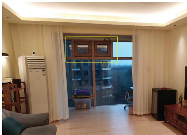
**Figure 23.** The openable area of the window is very small in a local passive house for experiments.
