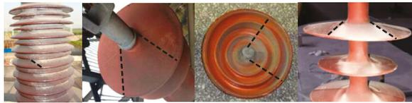
**Figure 1.** Non-uniform pollution between windward and leeward sides on insulator surface.
